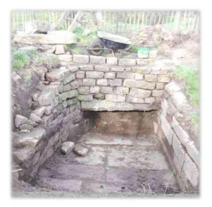
To ensure health and safety we erected chestnut pailing given the depth of the mill race. The Parish Lengthsman Tim Hoyles and Pilling's Parish Lengthsman, Graham Armer worked together to reconstruct the walls of the mill race and sluice gate with the stones which had been revealed and a few that had been put away for safe keeping.
